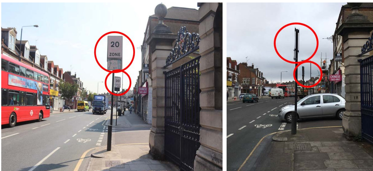
Figure 22 – Location where speed signs were rectified, before (left) and after (right) rectification
